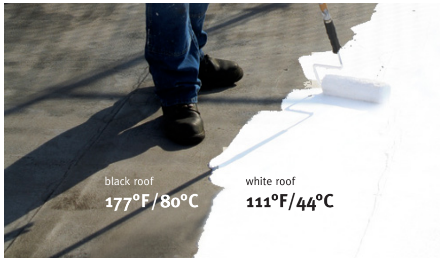
White roofs stay much cooler in the summer sun than black roofs. Shown above is an example of that difference on a day when the air temperature is 98°/36°C. Source: Data adapted from LBNL.
