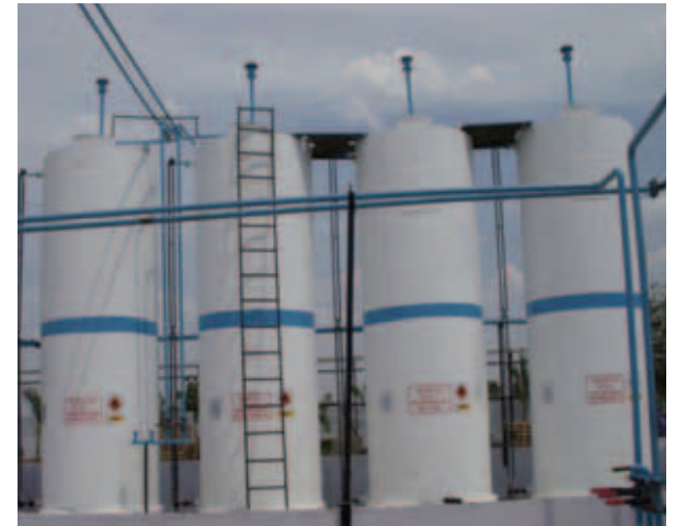
After Coating MS Tank
