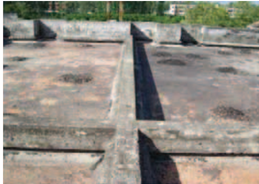
After Scraping of Bitumen
