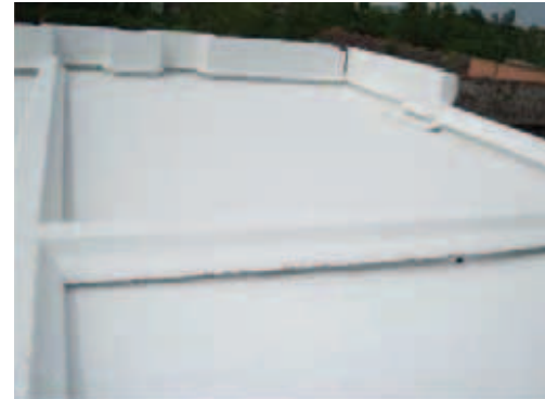
After Cool Roof Coating
