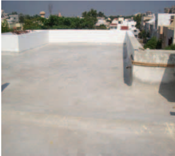
Before Coating Roof Area
