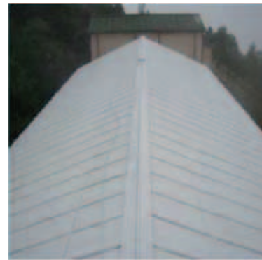
After Cool Roof Coating
