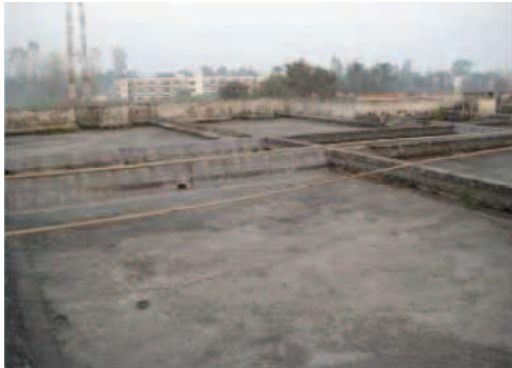
Surface before coating & treatment - Pantnagar
