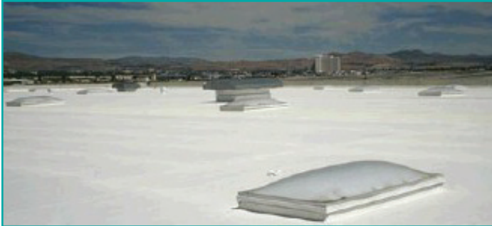
Figure 4: Single-Ply Membrane Cool Roof
