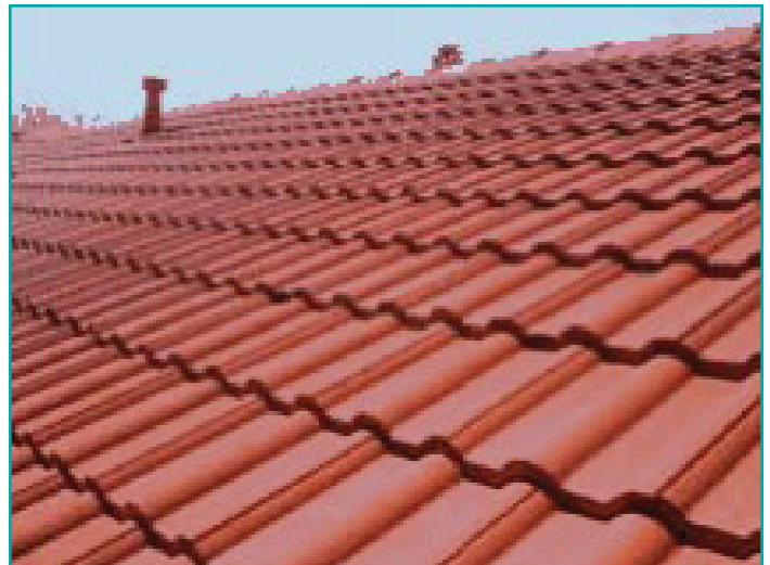
Figure 7: Thermoplastic Coating Cool Roof
