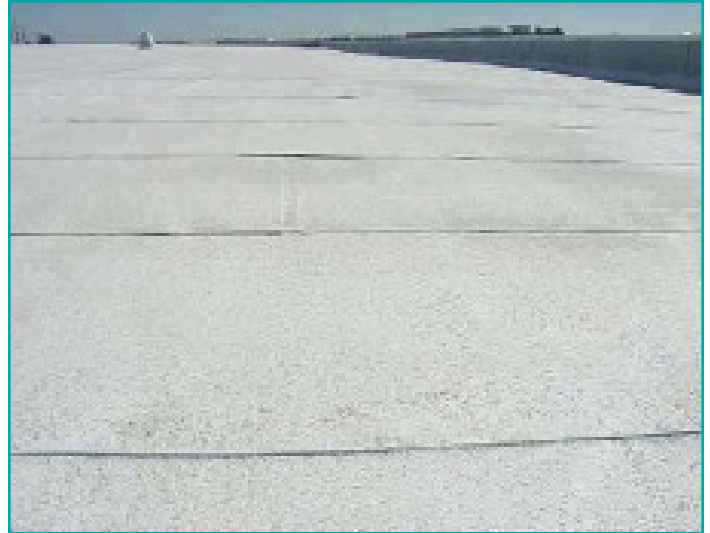
Figure 6: Cementitious Coating Cool Roof
