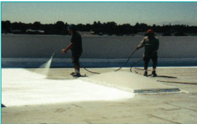
Figure 5: Typical Cool Roof Spray Installation
