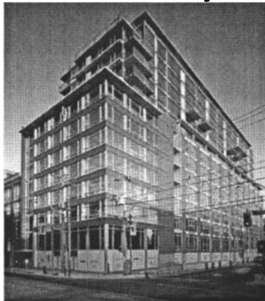
High Density Case-Study Building
