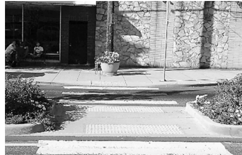
'Domes', being tested at SW Woodstock, are intended to assist visually-impaired pedestrians.
