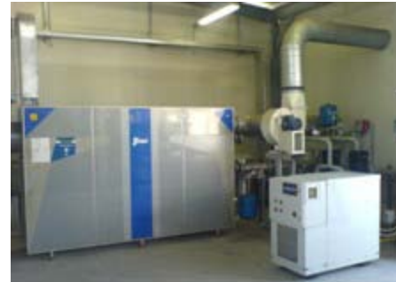
Gas CHP Microturbine
