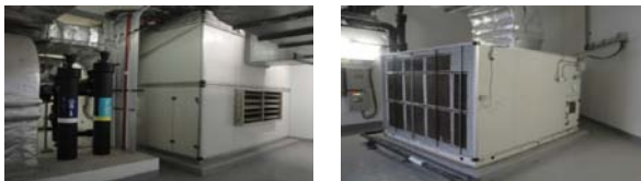
Picture 15 - Wheel air-to-air heat exchangers are installed.
