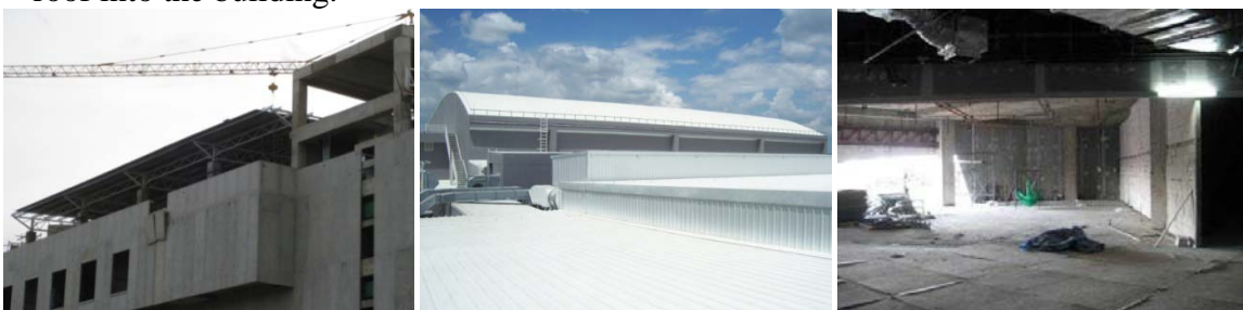
Picture 24 - walls and roof of the building
