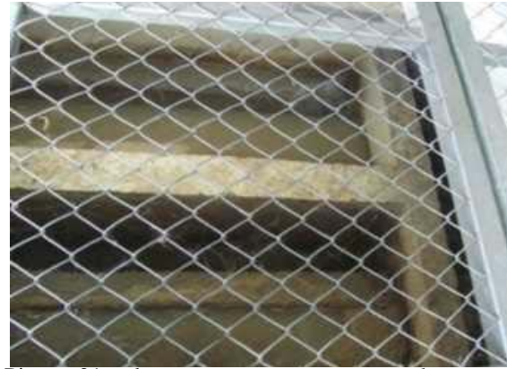
Picture 21 - the waste water treatment ponds, grease traps and trap debris
