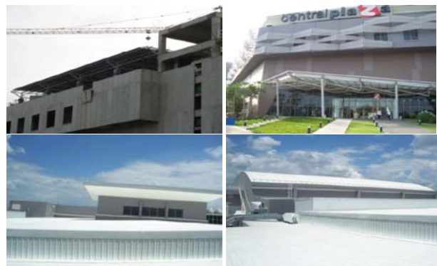
Picture 26– wall and roof
