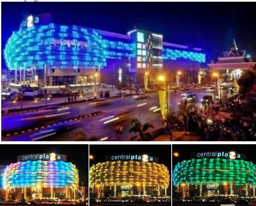
Picture 30– outdoor LED lighting system and be color changed at night.
