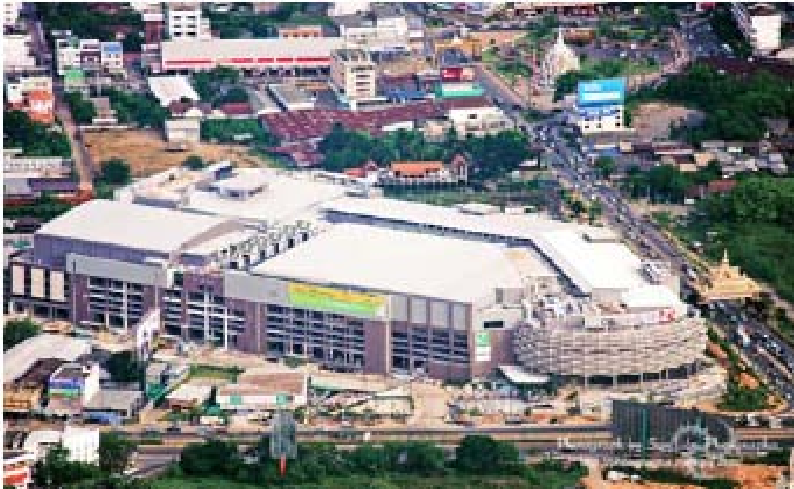
Picture 28 – Rooftop and building view from sky
