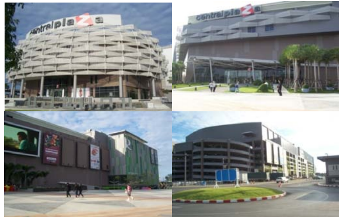
Picture 25– 4 side views of the building
