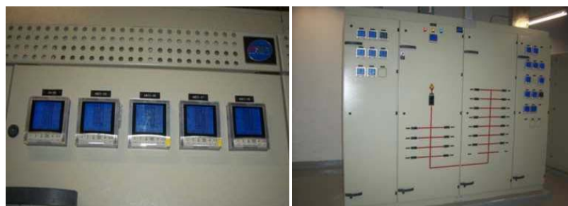
Picture 34 – energy meters monitoring energy consumption in lighting and air conditioning in various zones
