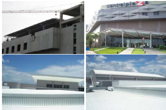
Picture 47 - Wall and Roof
