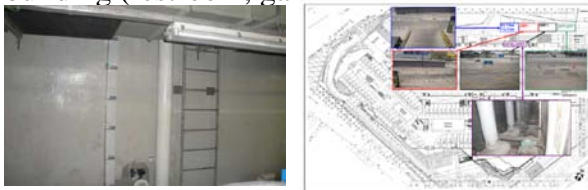
Picture 20- water storage tank
