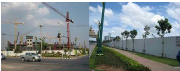
Picture 40 - wall around the construction area during the construction.
