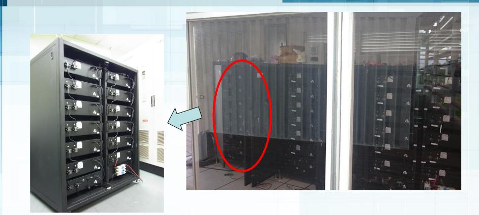
633V, 85Ah (53 kWh) per cabinet Total energy storage is three cabinets containing 159kWh.
