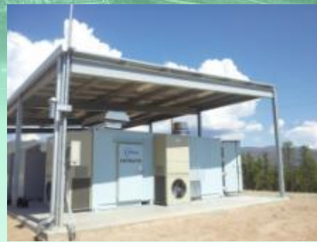
PCS (Direct current \rightarrow Alternating current)
