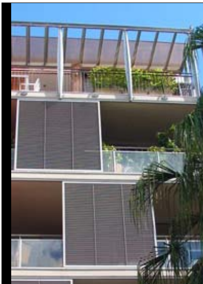
Use of balconies and louvers
