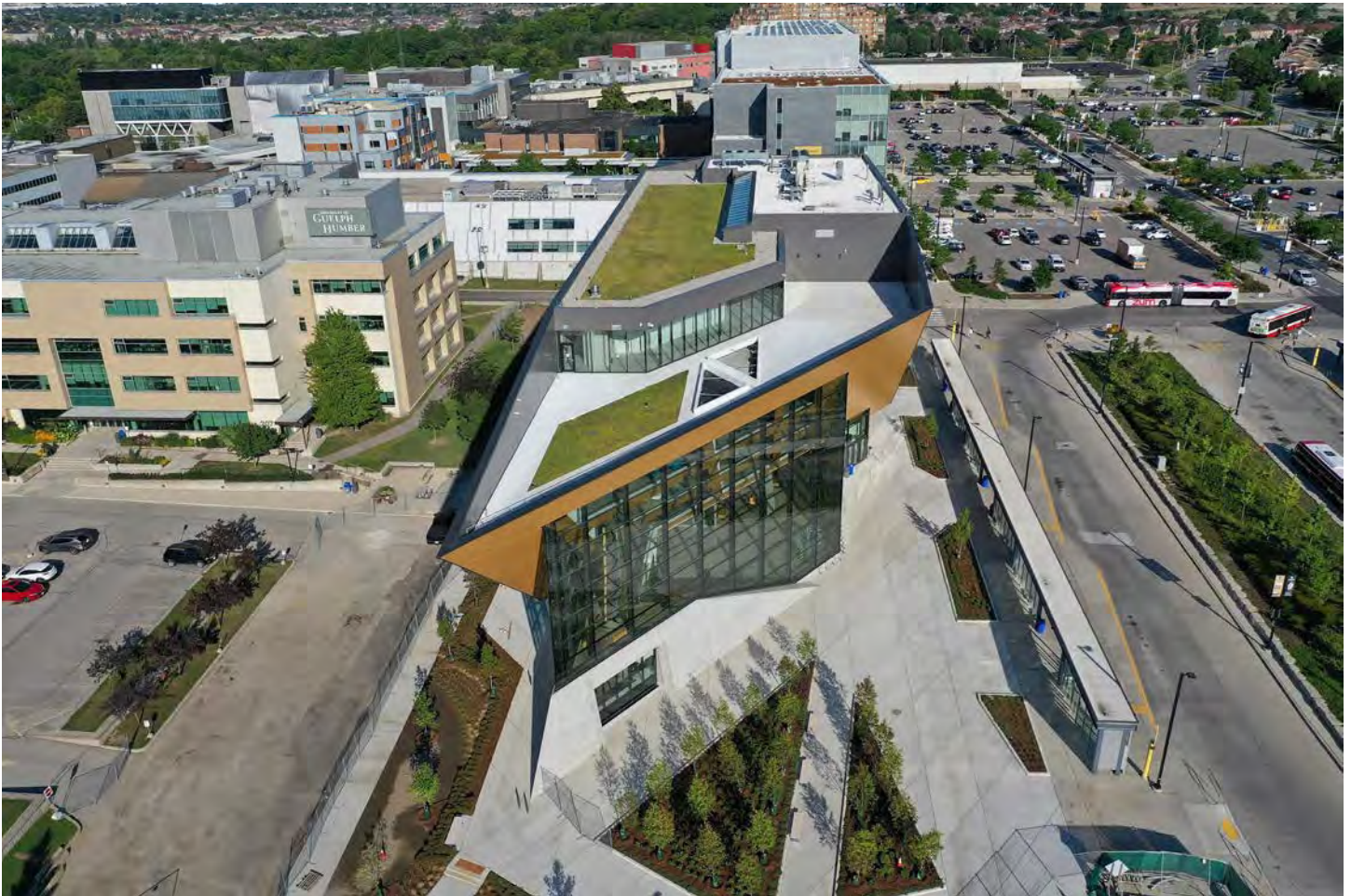
Above: A green roof on the 5th floor roof contributes to water retention on site.
